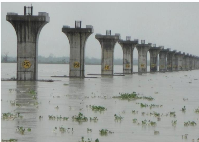
Fig 1: Series of piers with reinforcement for seismic arrester
