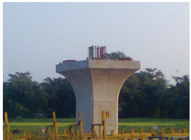
Fig 2: A single pier with seismic arrester re-bars
